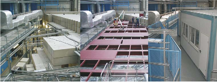
FIGURE 7.4 Photographs taken from the same position in the ESR Experimental Hall and showing the construction of the HITRAP platform. Left: situation in 2004 before construction. Middle: situation in 2005 when the platform was erected for the huts housing the electronics of the HITRAP facility and of the HITRAP experiments, for RF power supplies and other devices. Right panel: situation in 2006 when the platform is ready, the huts are in place, and the installations are almost completed.
